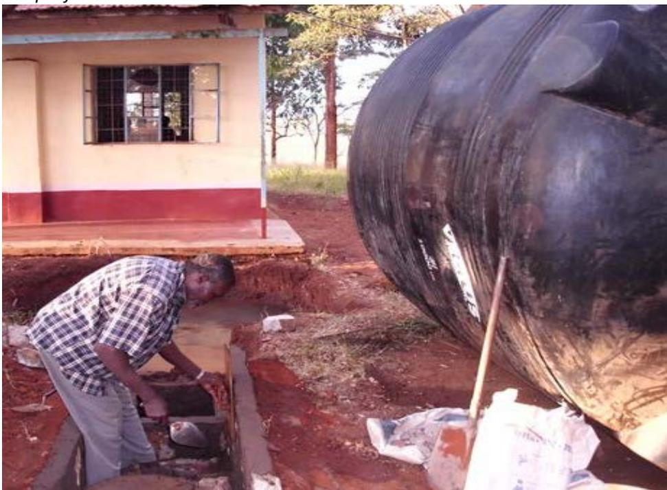
*Construction of the base for water tank*
