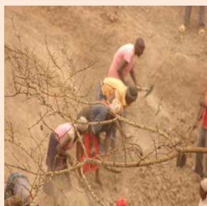
Construction of sand dam in Kalama
